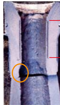
Erosion only below the carbon-free lined area
